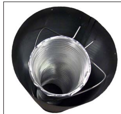
Figure 20: Wire Spacer in Place.
