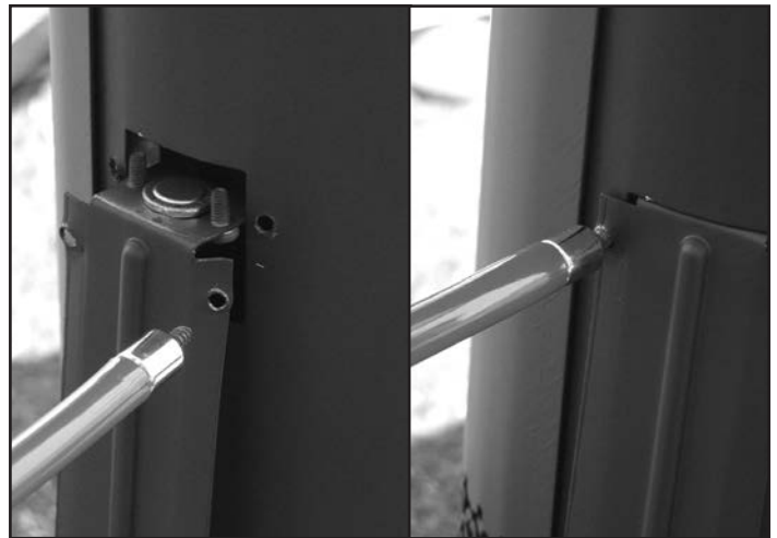
Figure 49: Spill switch installation.
