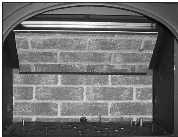
Figure 64: Back brick panel in place.
